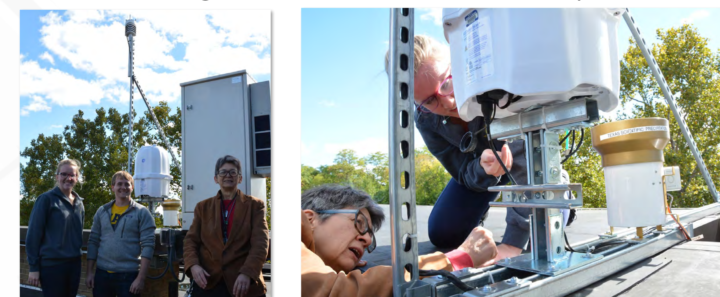
Travis Smith and Rebecca Lynch (CVT undergraduate fellows) with Prof. Kim Kearfott (CVT Thrust Area 6 Lead) installing radiation detectors and weather monitoring equipment on the Cooley building roof-top at UM
