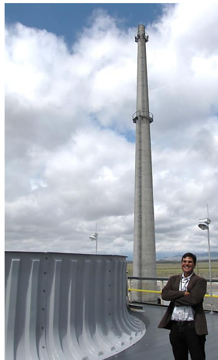
Colling fan duct and the exhaust stack at ATR
