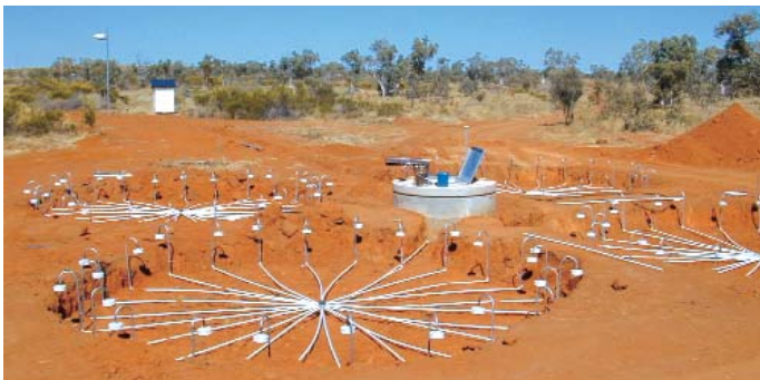
Fig. 2. Partially installed infrasound site in Warramunga, Australia. The pipe rosette will be buried so that only the intakes (white “shower heads”) will be above ground and the four rosettes will be connected to the microbarometer located in the cement vault. (Photo by D. Christie).
